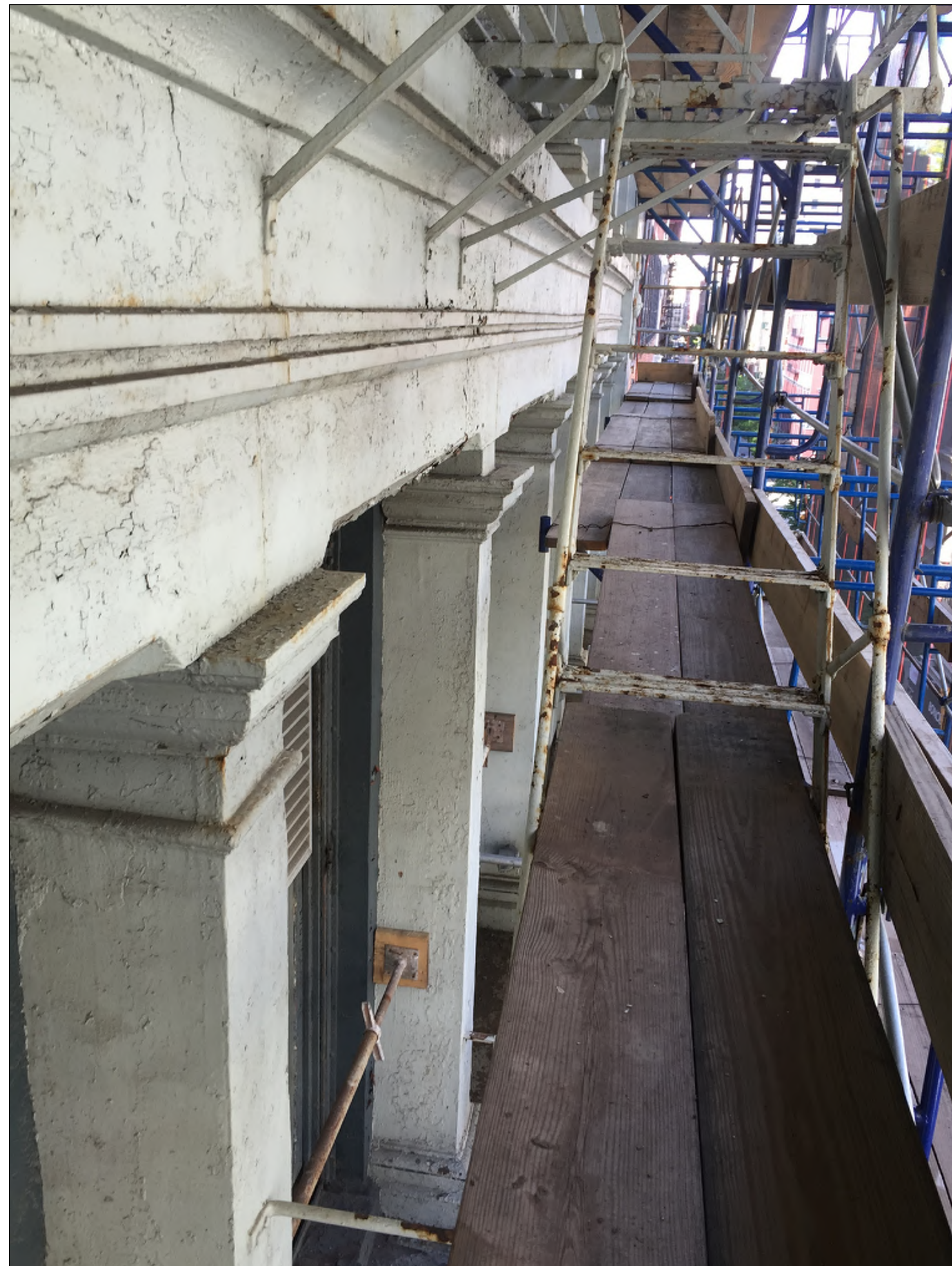
PRE-RESTORATION CAPITALS ON CROSBY FACADE
