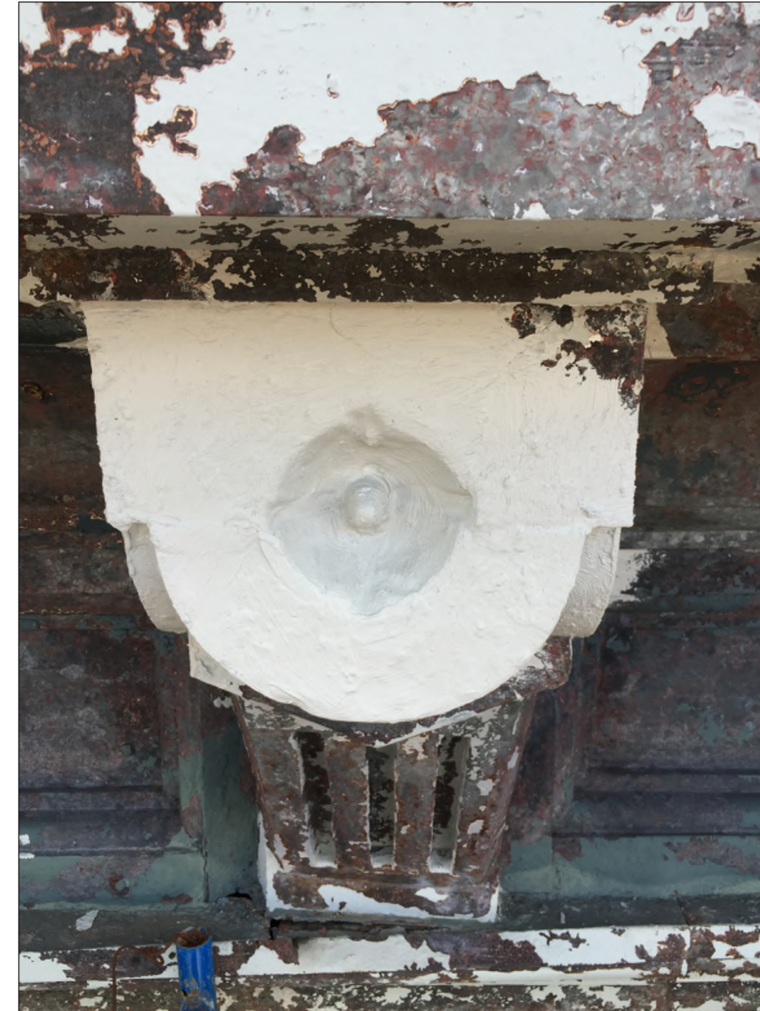
CORNICE IN PROGRESS OF RESTORATION
