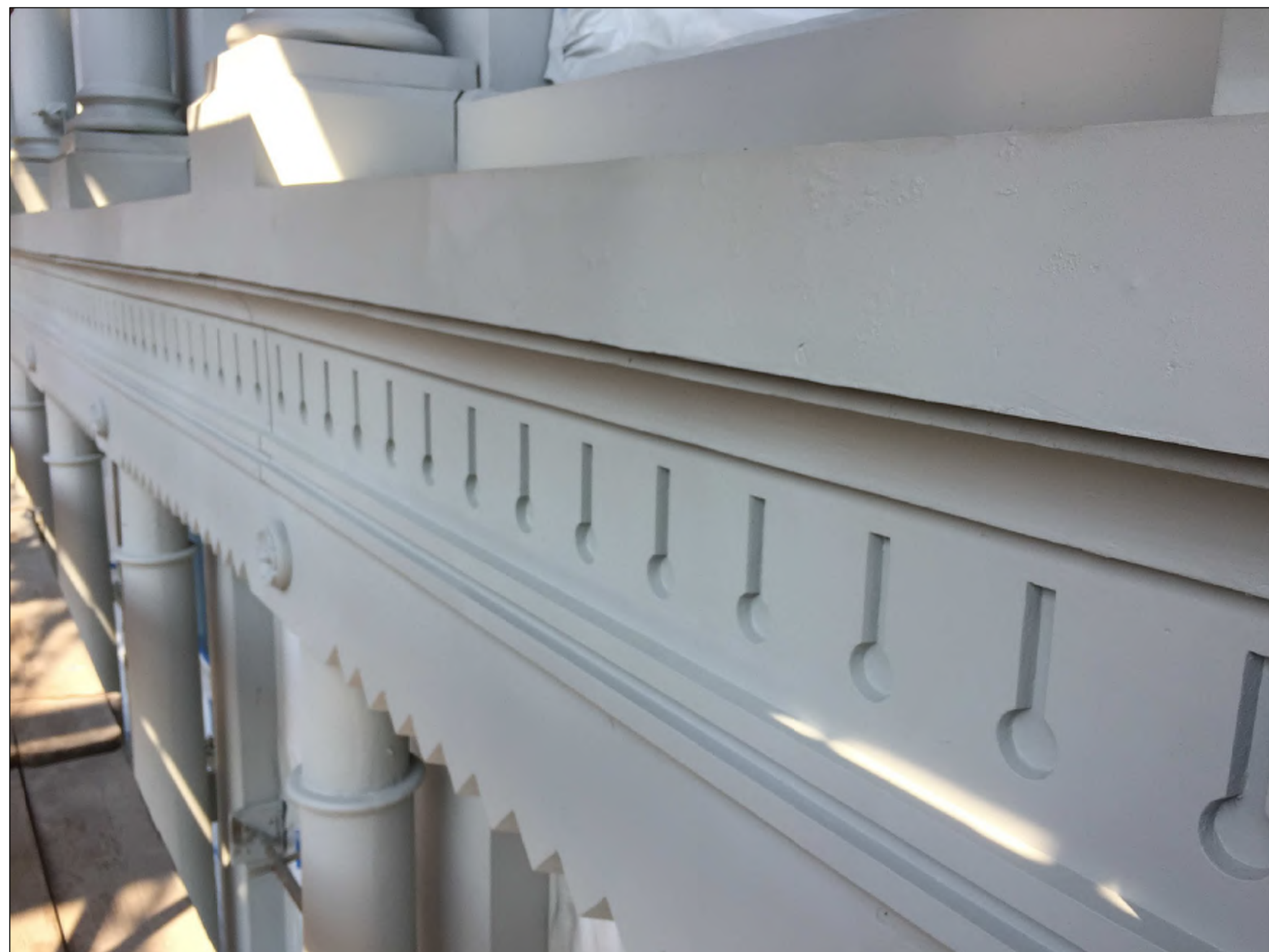
CAST IRON AFTER PAINT REPAIR
