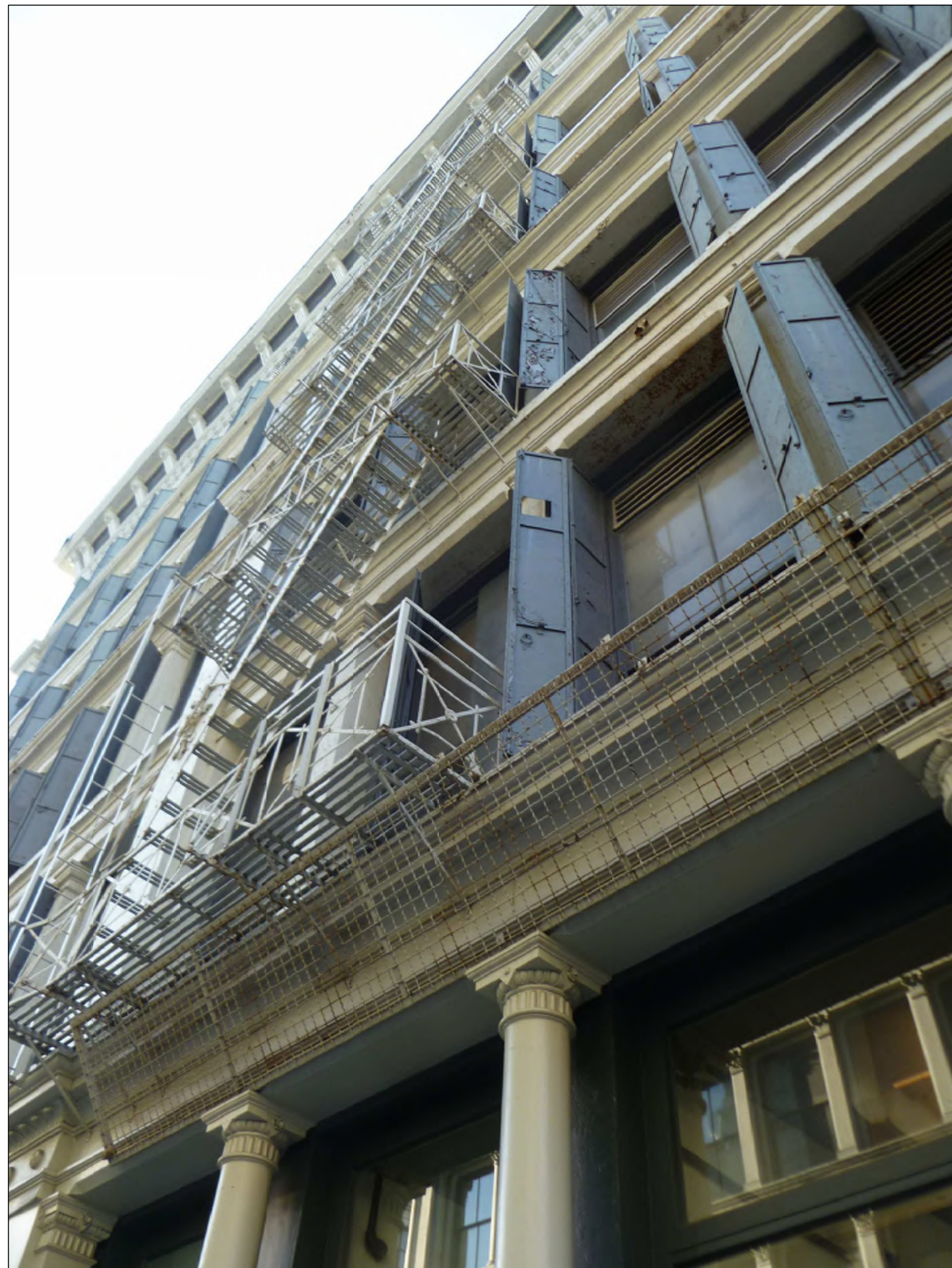
CROSBY STREET FACADE, EXISTING SHUTTER CONDITIONS.
