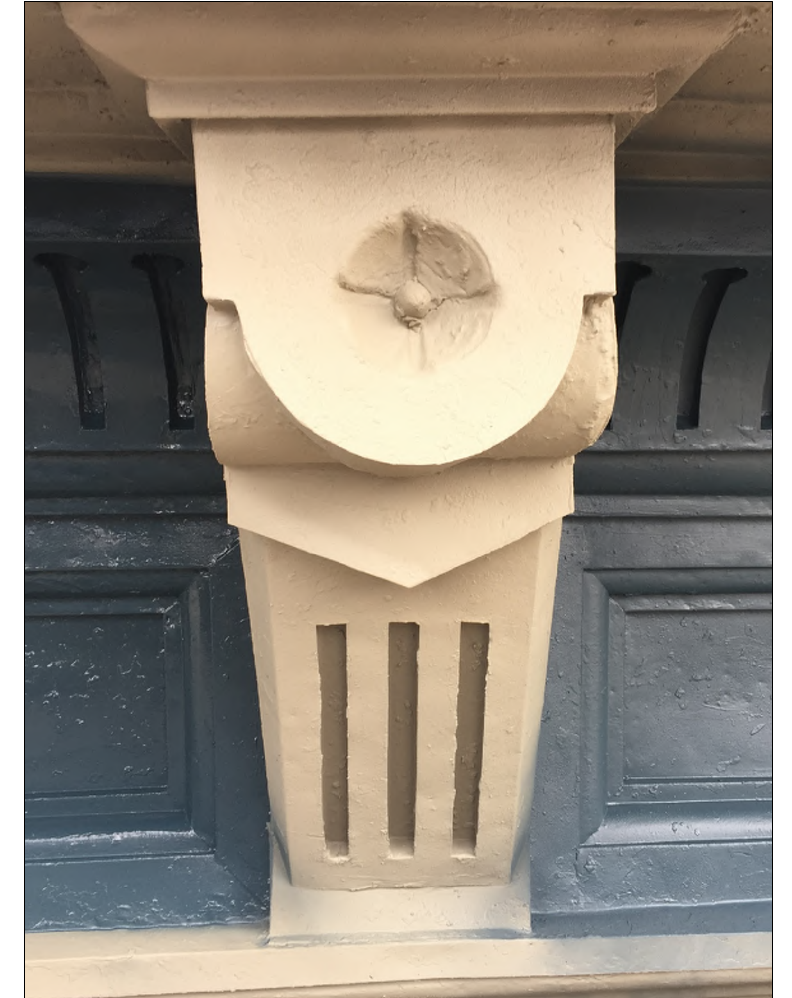
CORNICE CONDITION AFTER RESTORATION PRIOR TO TOP COAT
