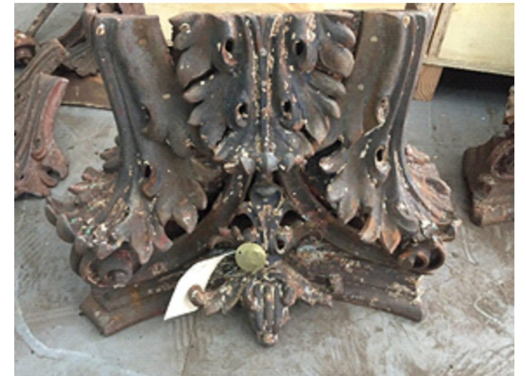
REMOVED CAPITAL DURING INSPECTION SHOWING TAGGING SYSTEM
