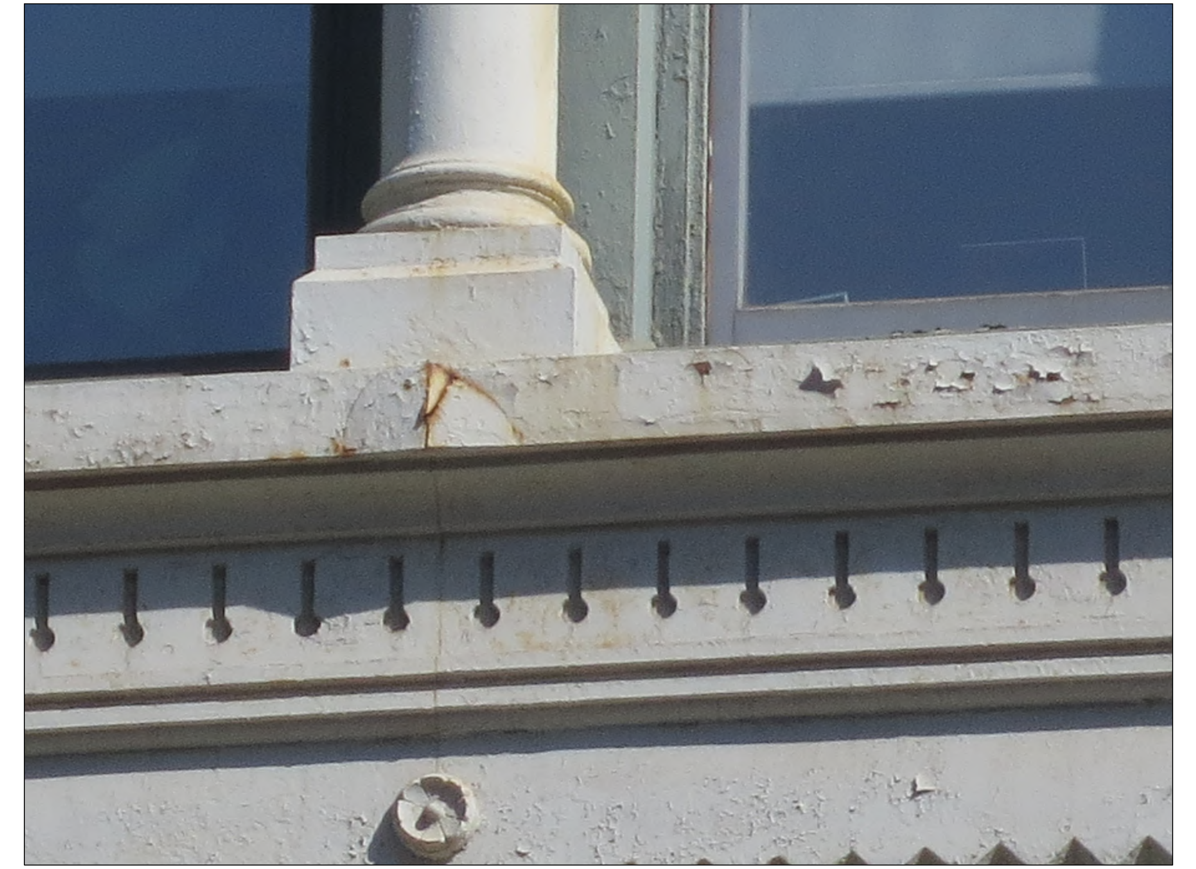
WINDOW SILL & CAST IRON CONDITIONS
