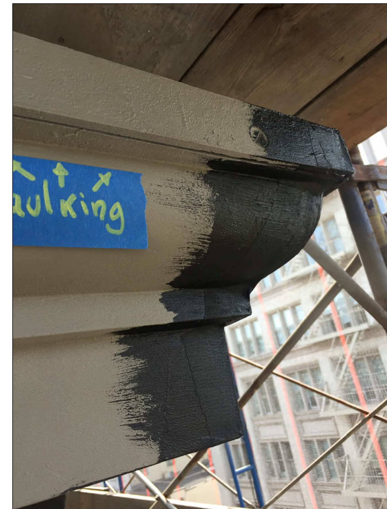
CORNICE DURING SECONDARY COATING
