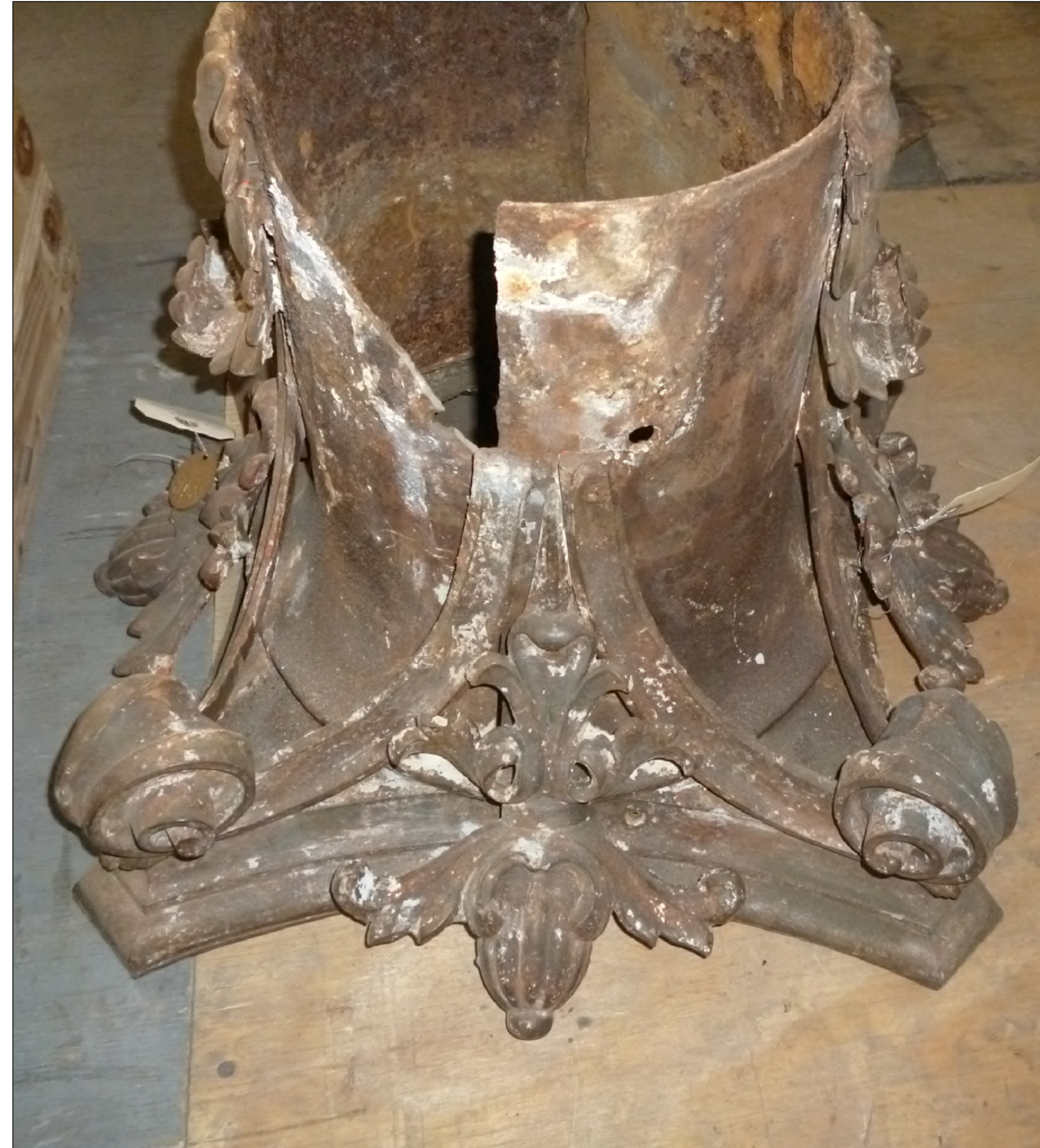
REMOVED CAPITAL SHOWING CRACKED BELL HOUSING
