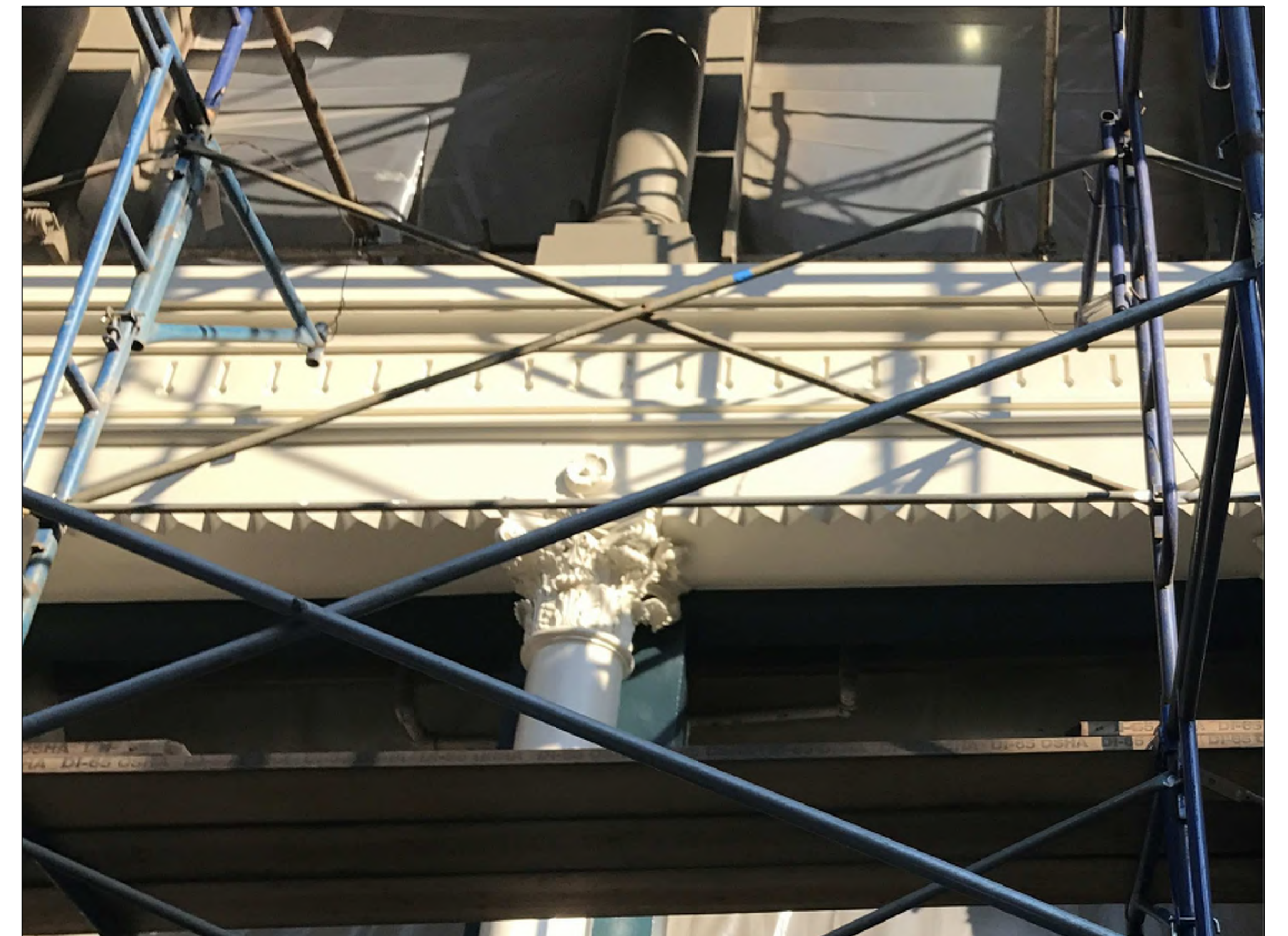
WATERPROOFING, SECONDARY AND TOP COAT FINISH PAINT
