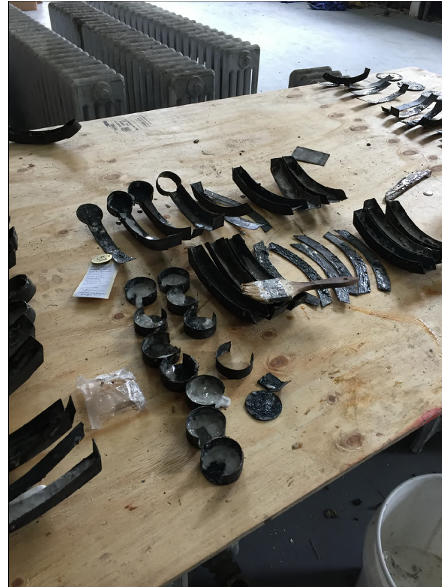
CORNICE COMPONENTS DURING RESTORATION
