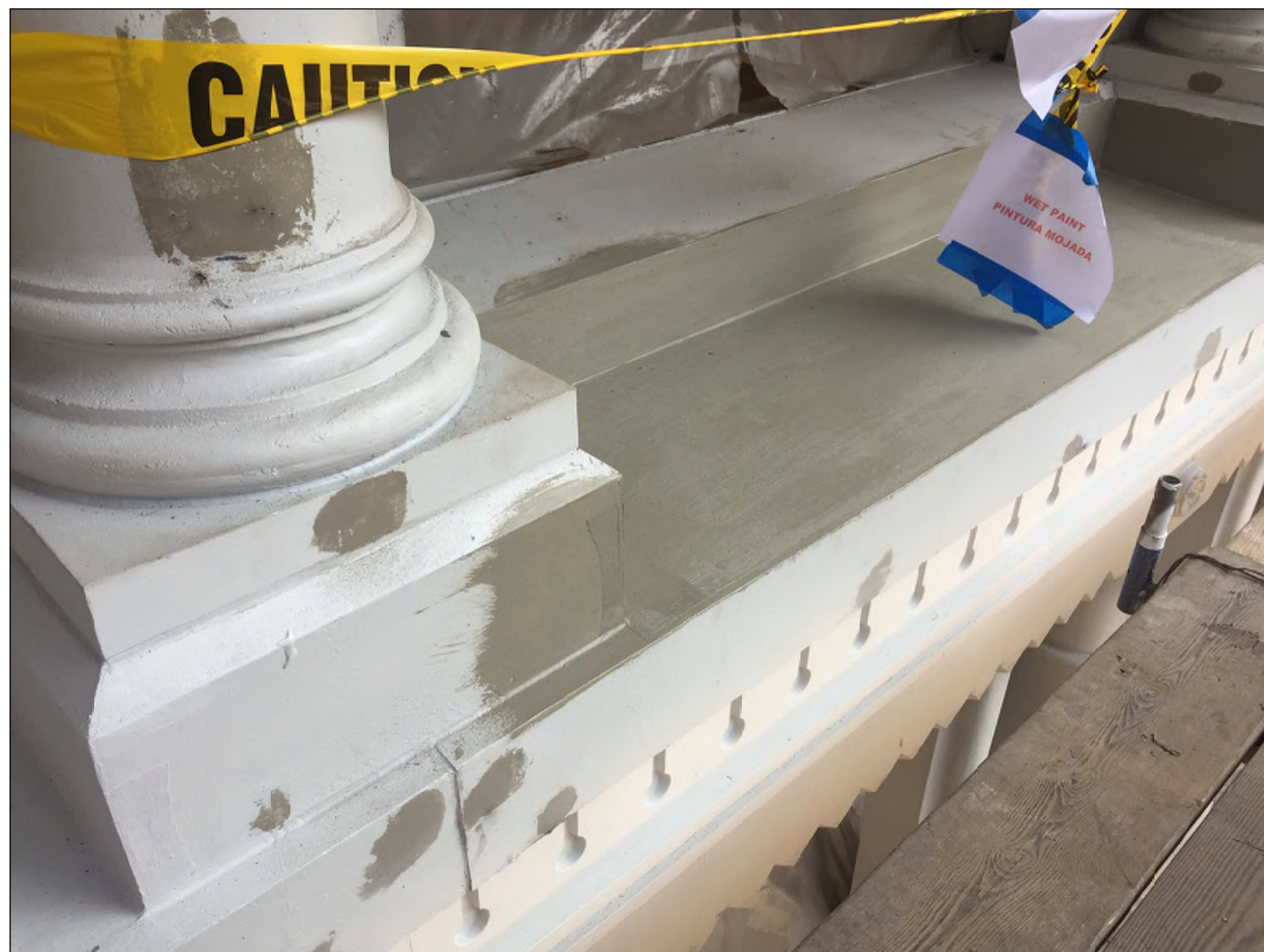
CAST IRON REPAIR AFTER PATCHING PRIOR TO FINAL PAINT.
