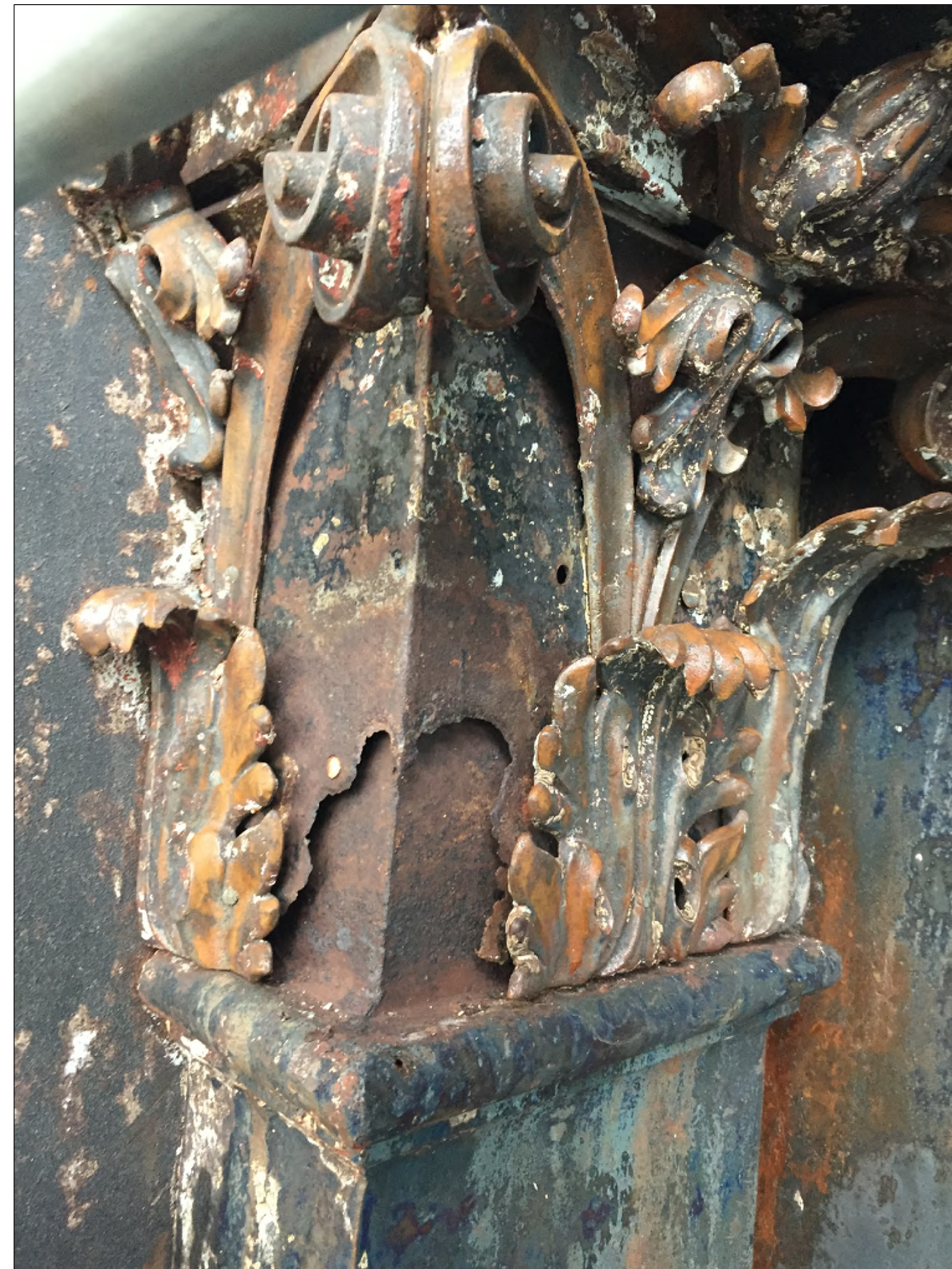
PRIOR TO REMOVAL SHOWING DETERIORATED BELL HOUSING
