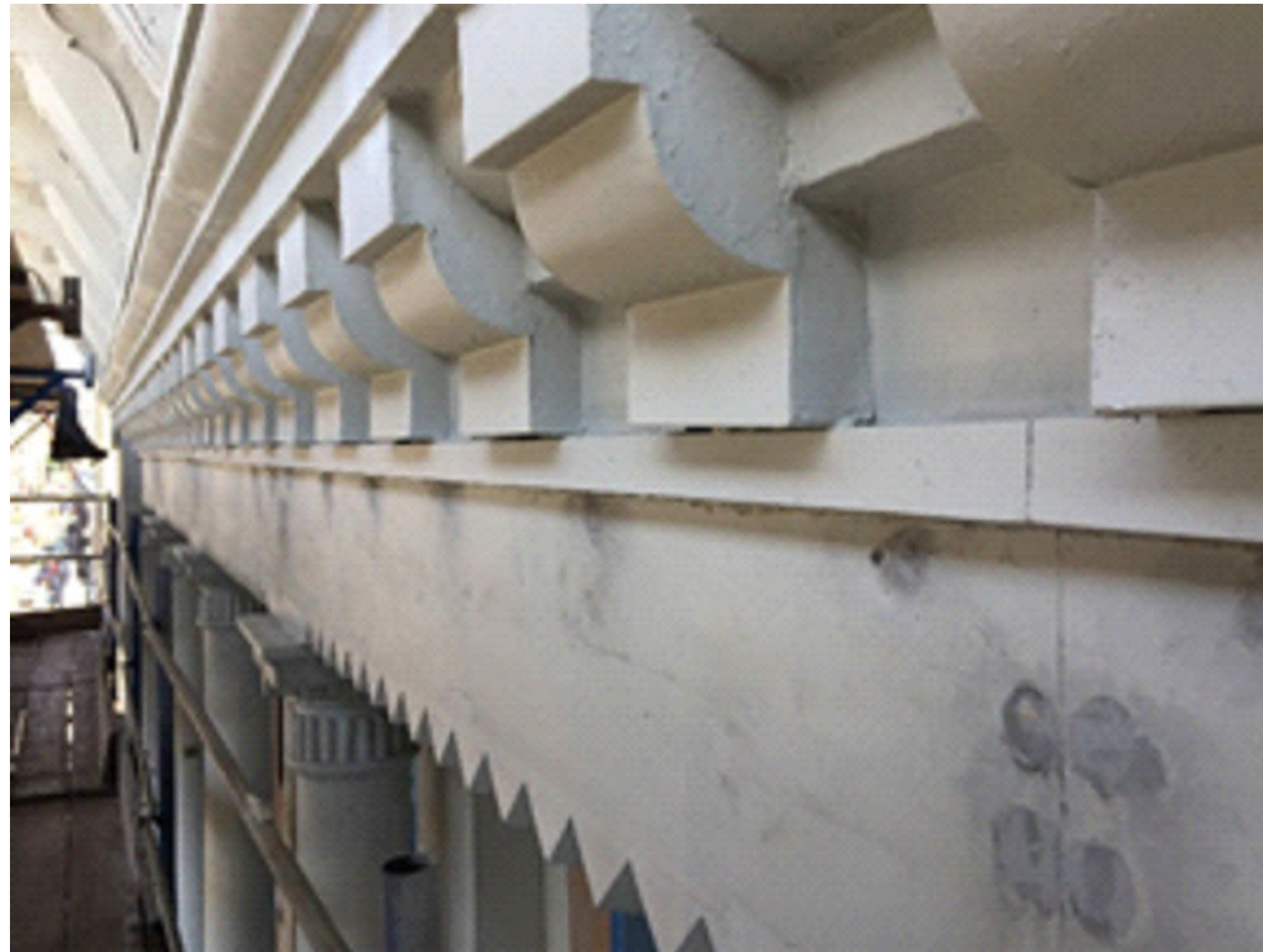
CAST IRON PATCHES PRIOR TO TOP COAT
