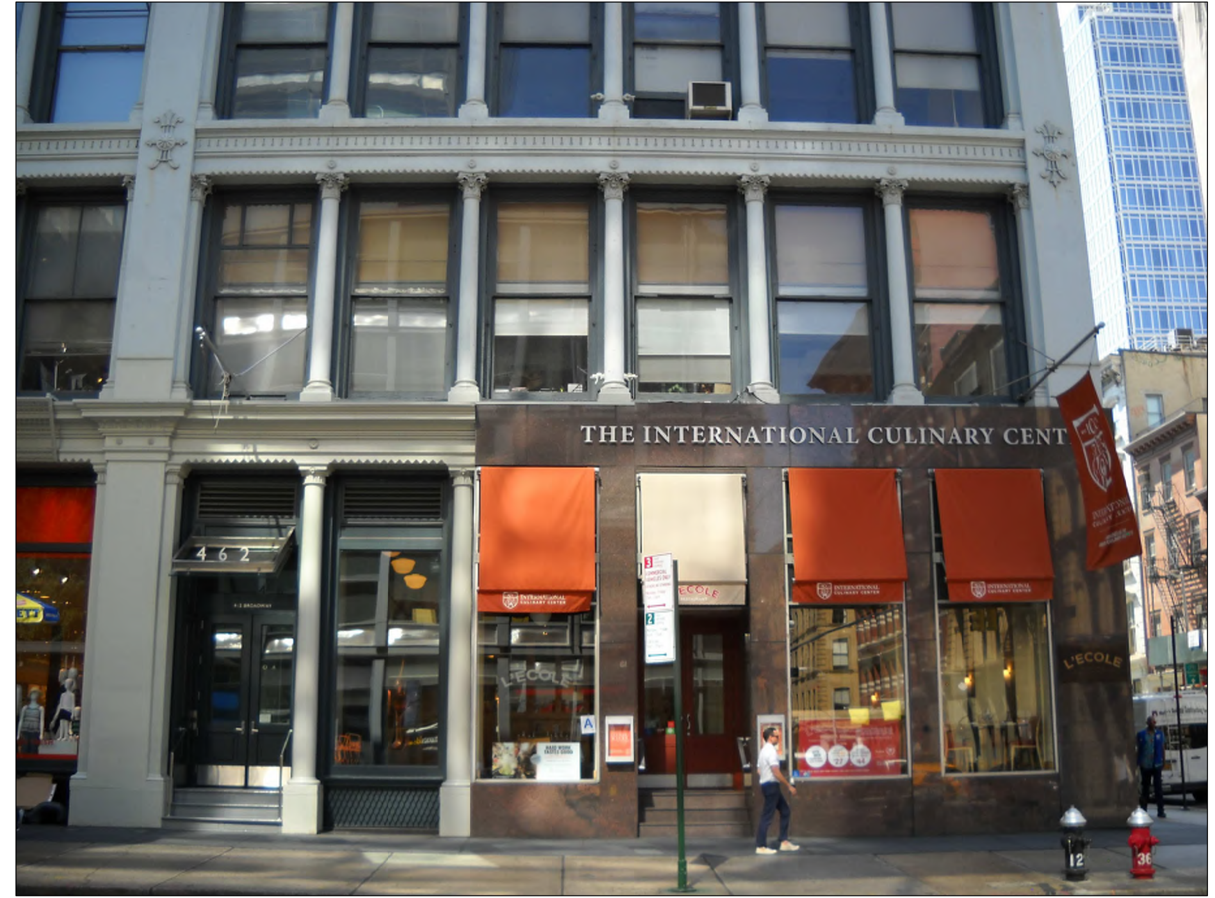
RECENTLY RESTORED BUILDING ENTRY & NON-HISTORIC STOREFRONT ON BROADWAY
