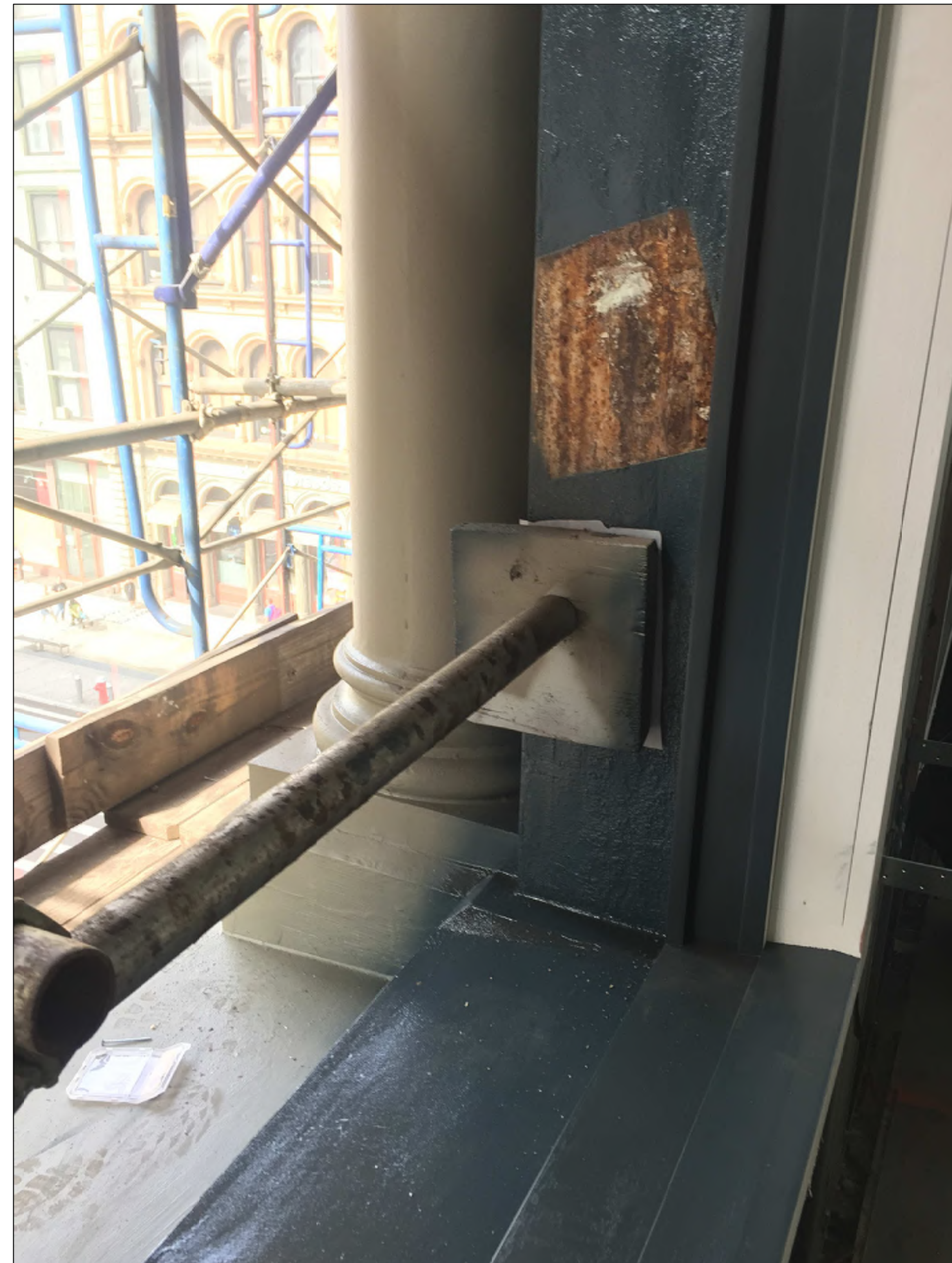
NEW WATERPROOFING AT CAST IRON SILL
