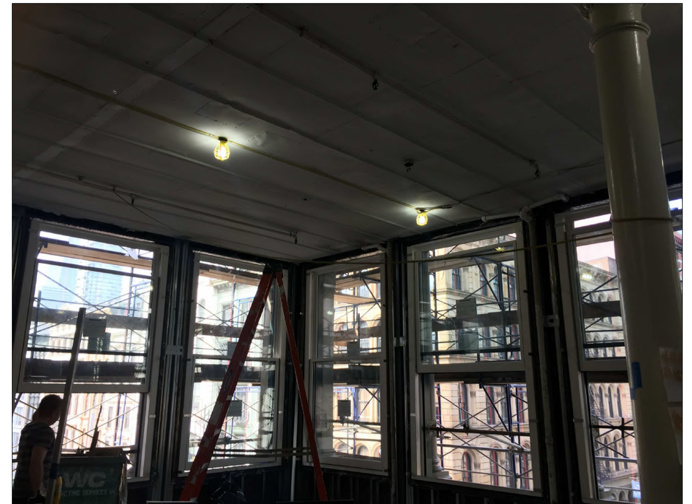
NEW WOOD WINDOWS INSTALLED
