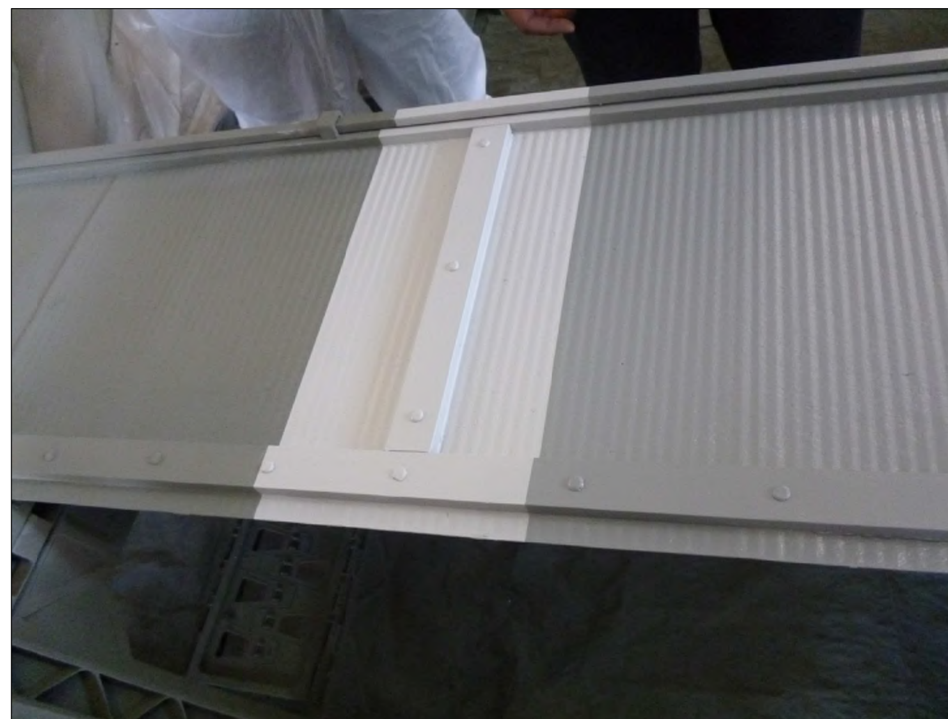
SHUTTER IN PROGRESS OF RESTORATION SECONDARY AND TOP COAT PAINT
