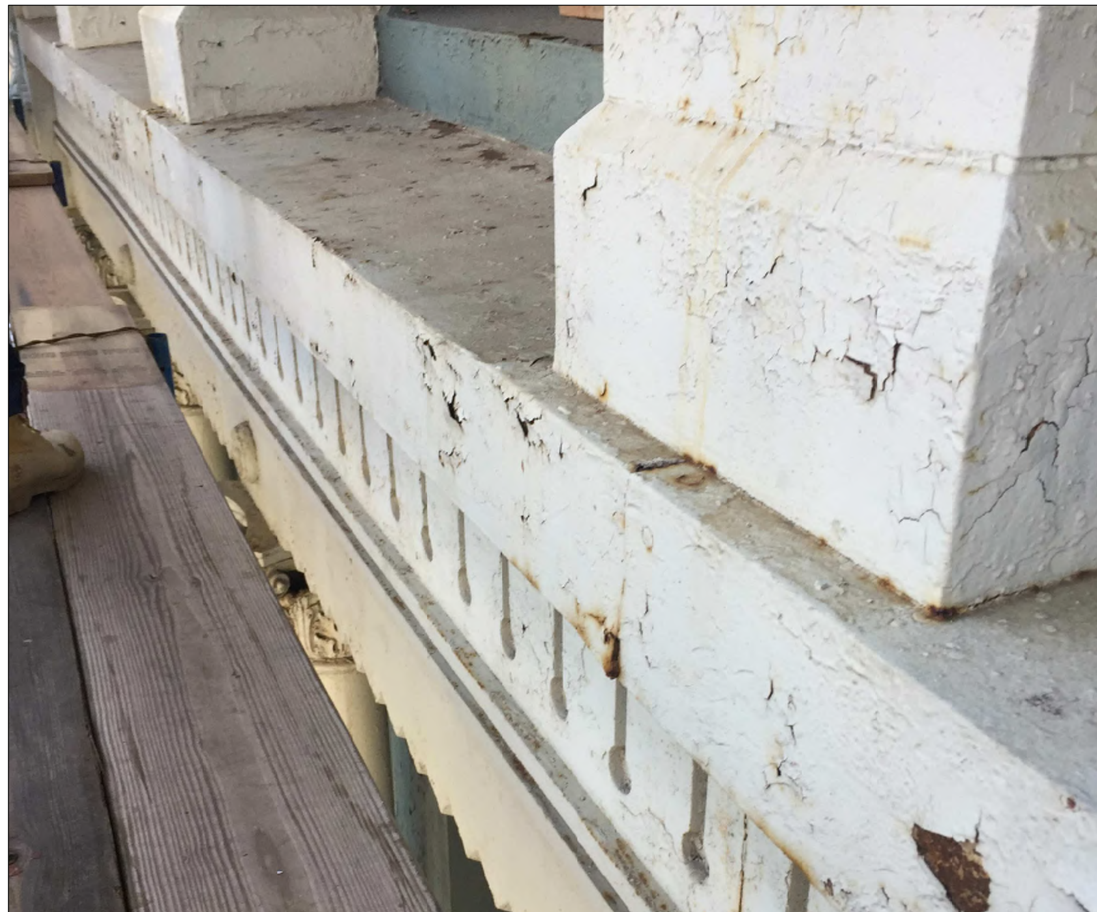
CAST IRON BEFORE PAINT REPAIR
