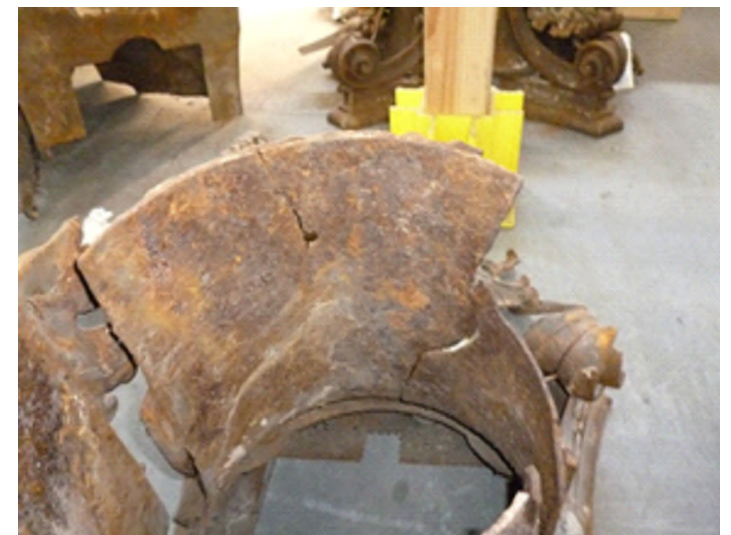
REMOVED CAPITAL SHOWING CRACKED BELL HOUSING
