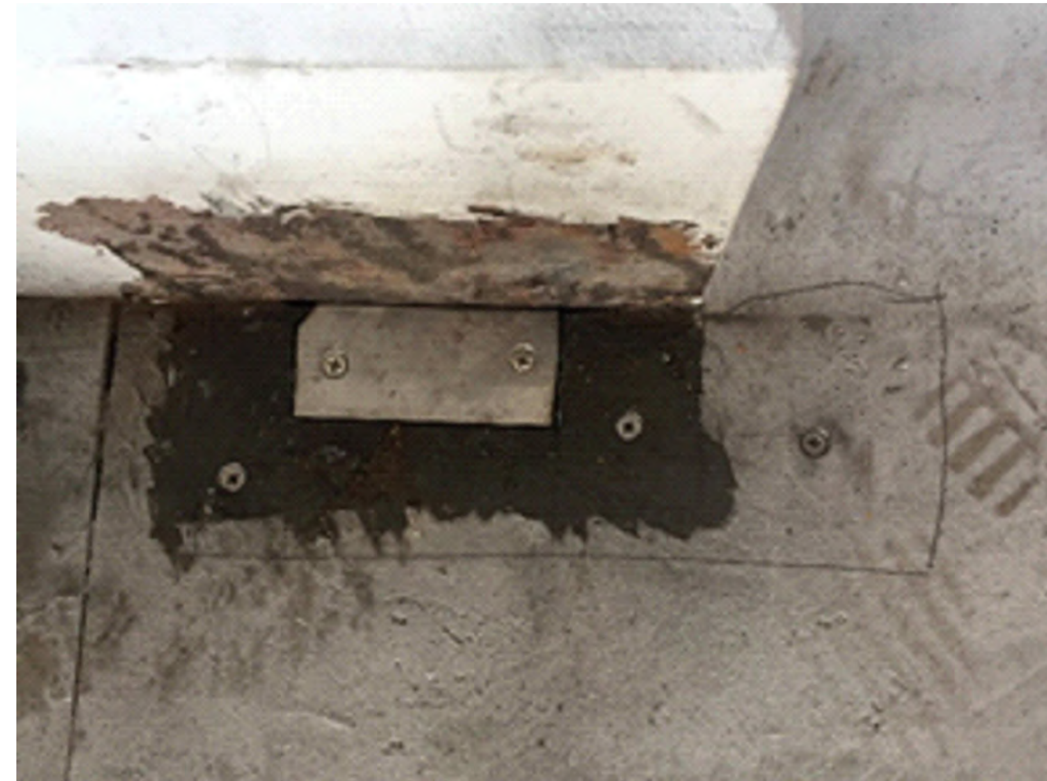
CAST IRON REPAIR - STAINLESS STEEL PLATE
