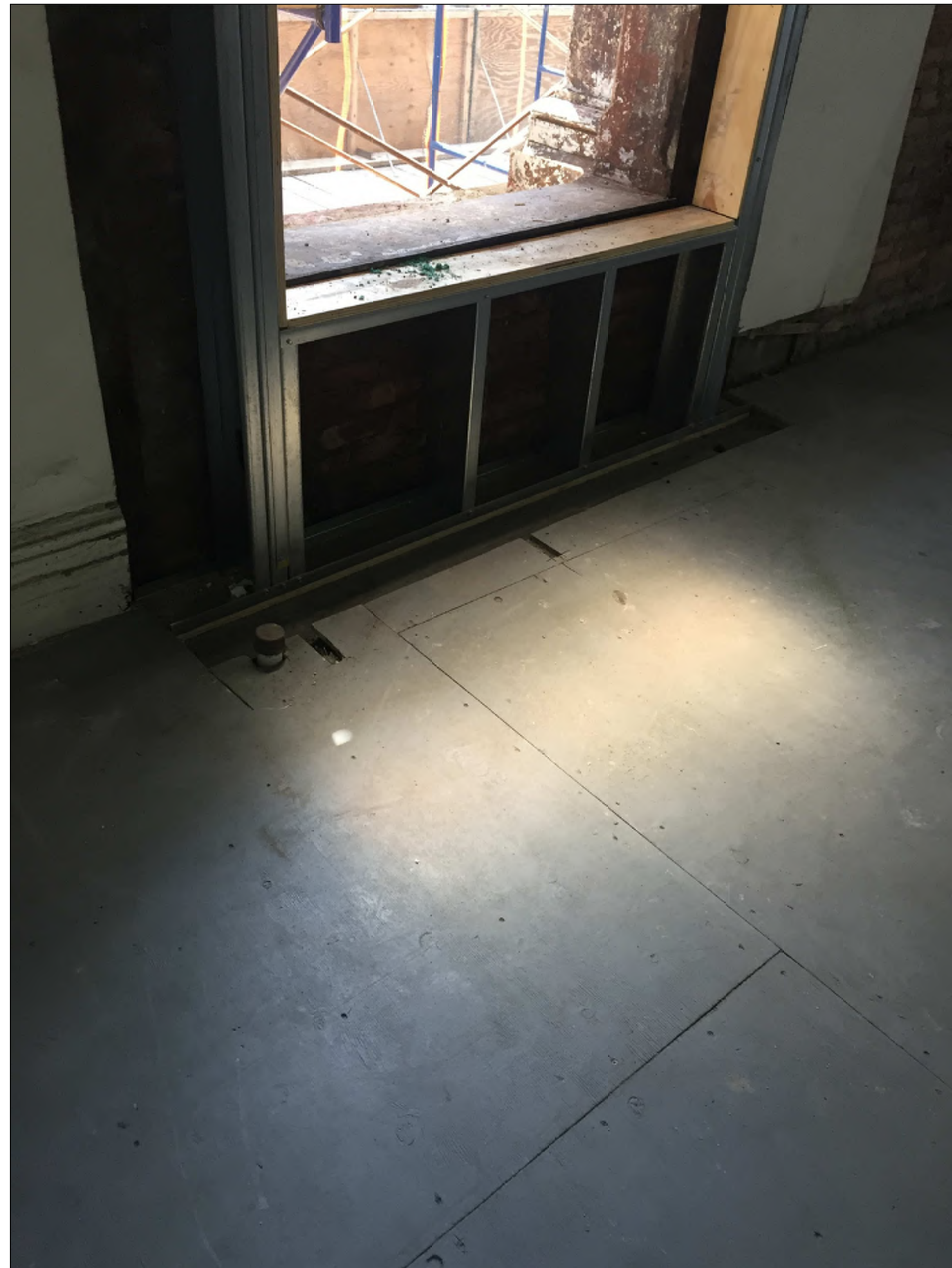
NEW FRAMING TO SUPPORT NEW WOOD WINDOWS
