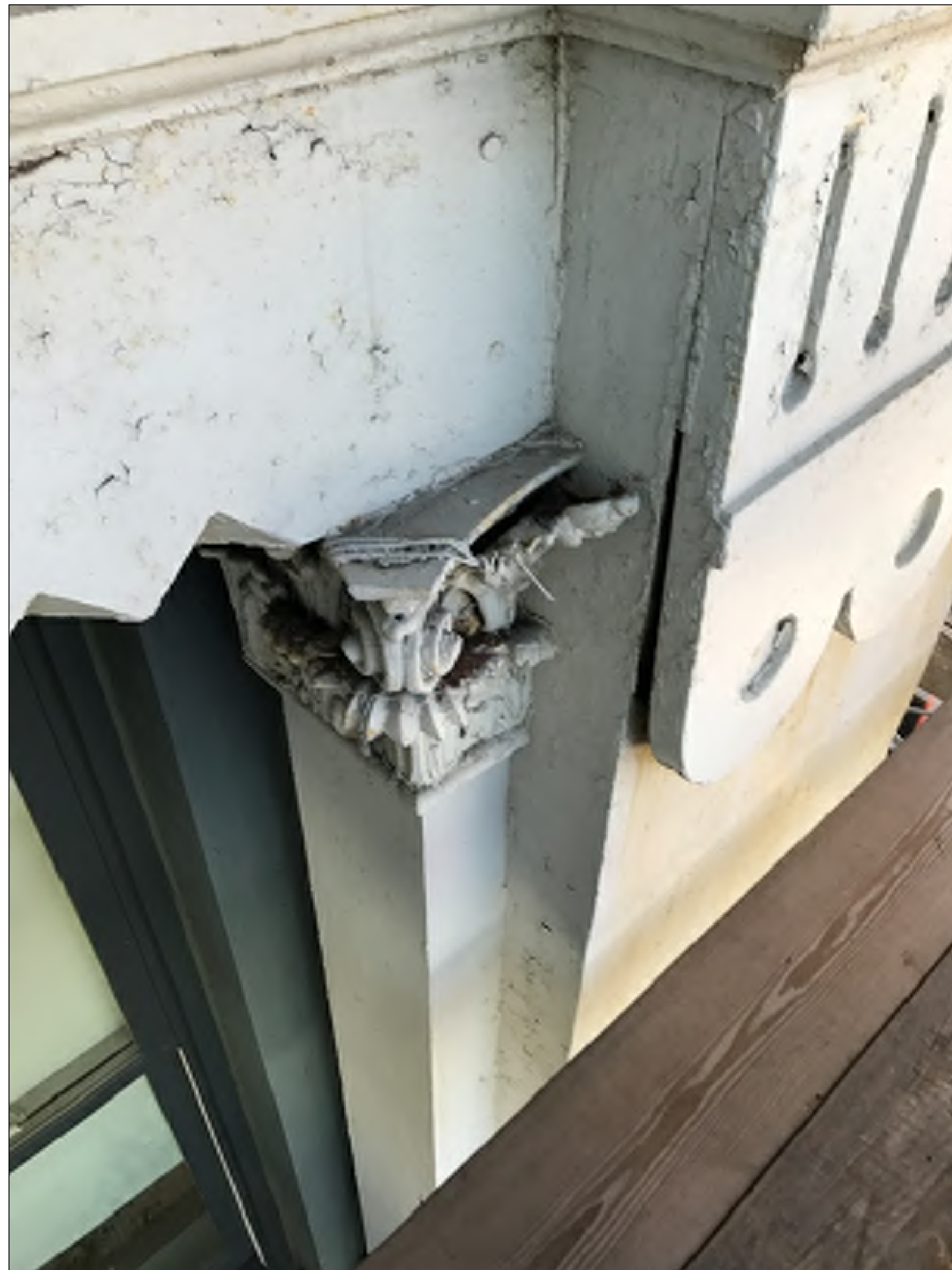
HALF SQUARE CAPITAL PRIOR TO REMOVAL
