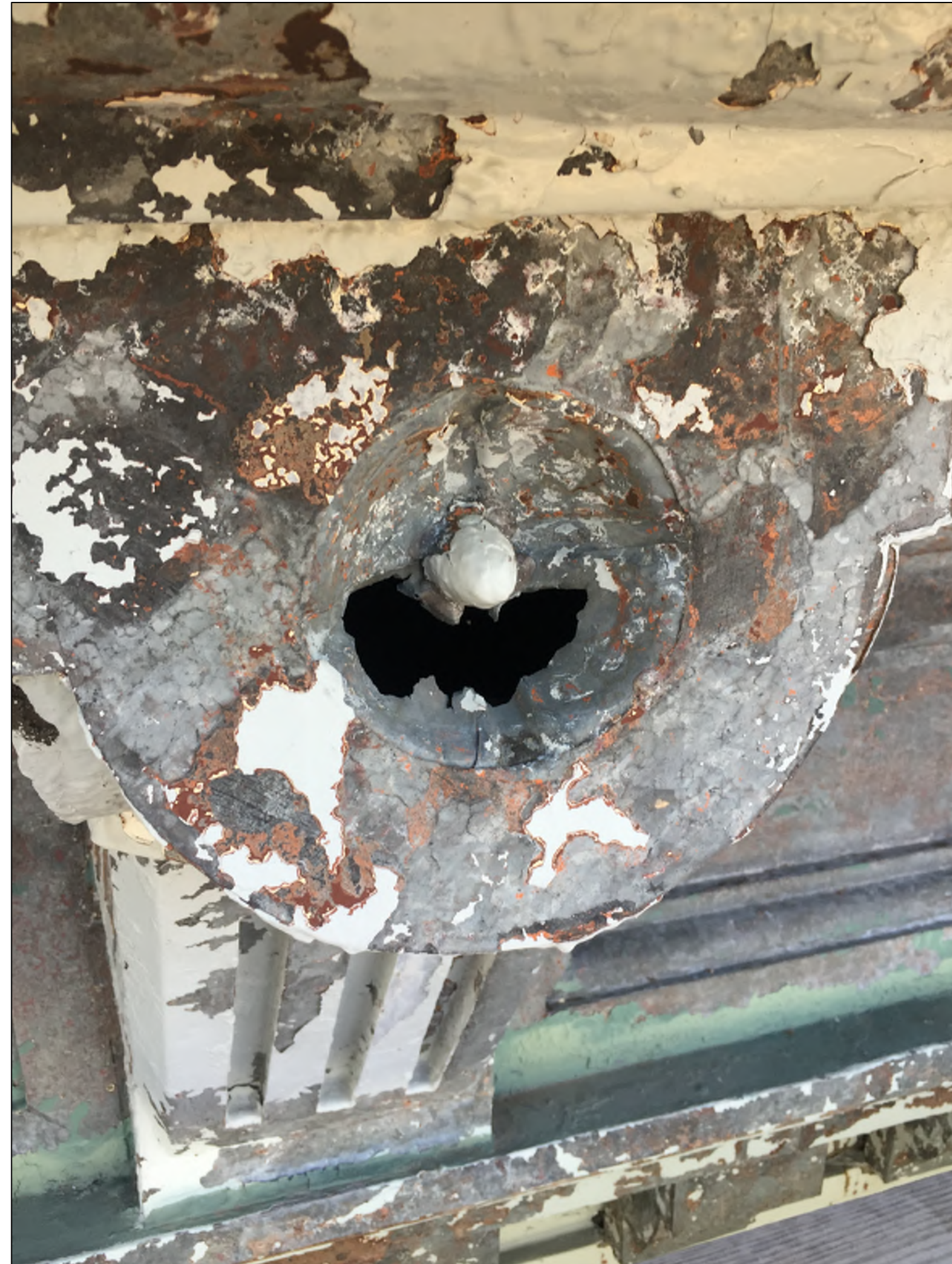
CORNICE CONDITIONS PRIOR TO REPAIR
