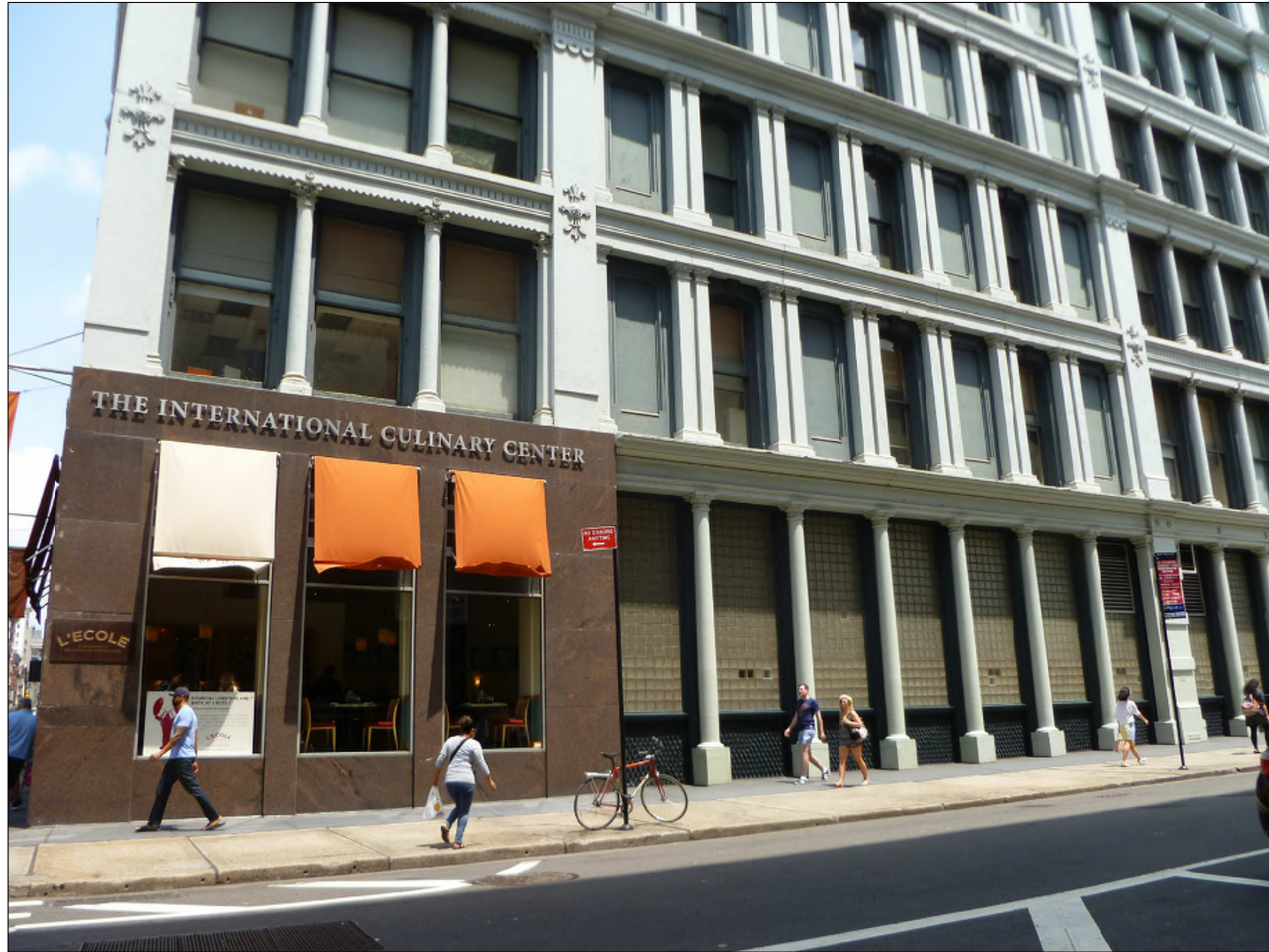
NON-HISTORIC STOREFRONT AT CORNER OF GRAND ST & BROADWAY
